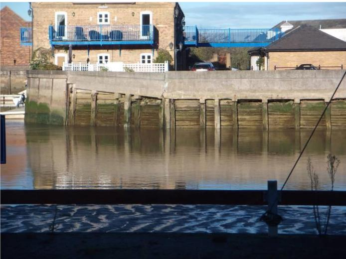
Our project consists of work to rejuvenate the failing flood wall and supporting quay along a 23 metre stretch of the River Chelmer. The damaged flood defence will be restored by installing new sheet piles in front of the existing wall and then a concrete infill section to form a strong composite flood wall structure. The existing standard of flood risk protection will be maintained throughout the works.
